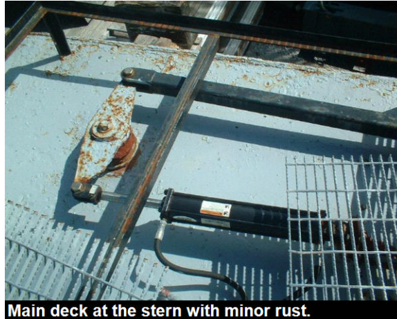
Main deck at the stern with minor rust.
